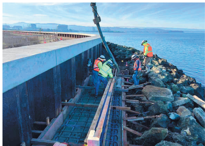
Concrete being poured into newly reinforced levee and sea wall as part of the Levee Improvements Project.
