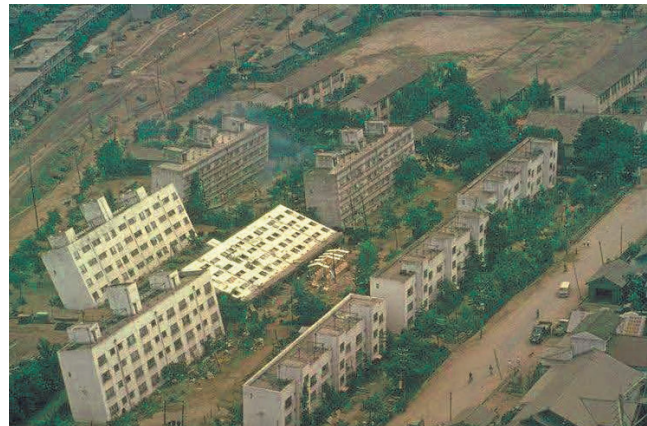
Liquefaction during the 1964 Niigata Earthquake
