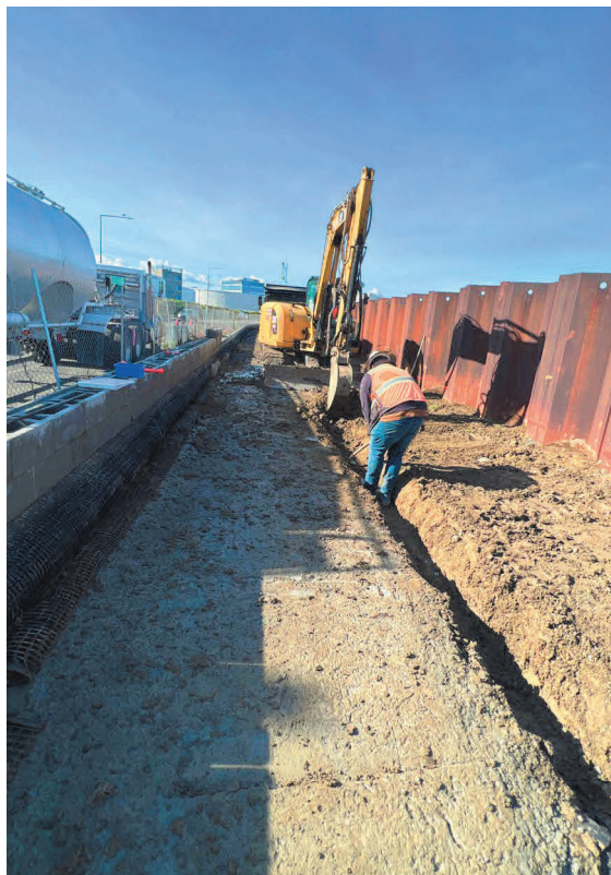
Levee retaining wall under construction
